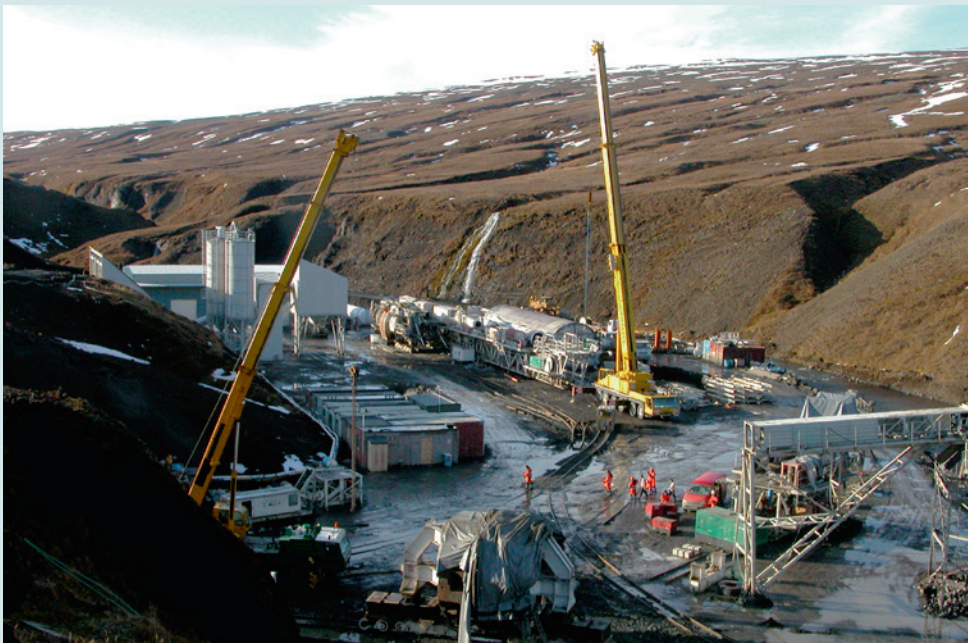
Figure 20 — Work site by one of the intake tunnels during the construction (top photograph) and the same area after clean-up (bottom photograph).
