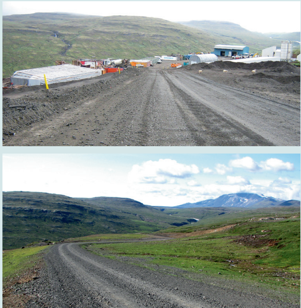
Figure 19 – The Impregilo premises during construction (top photograph) and after the clean-up (bottom photograph).
