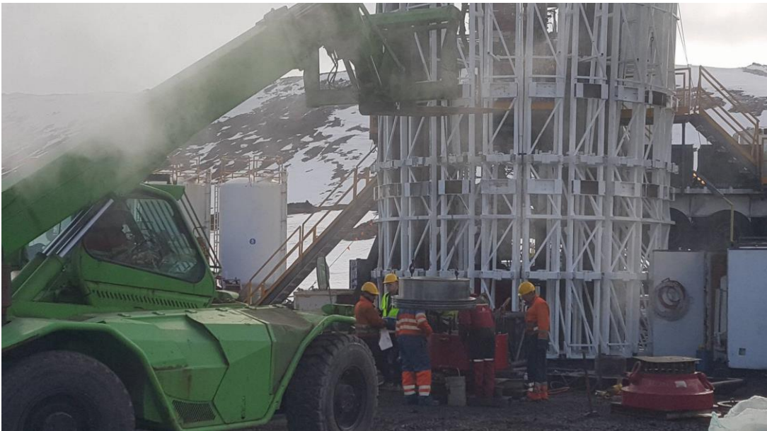
Figures 1-3. The drill crew working taking down the BOP.
