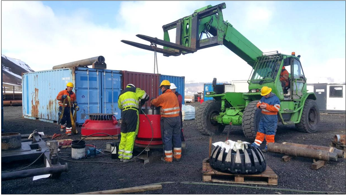
Figure 8. The drill crew at BG-11 working on repairing the lower annular BOP.
