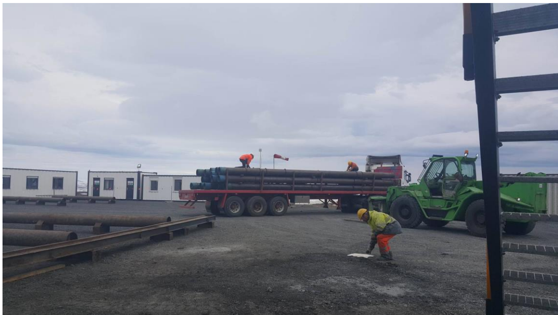
Figure 7. The 13 5/8 " anchor casing being transported to the drill site.
