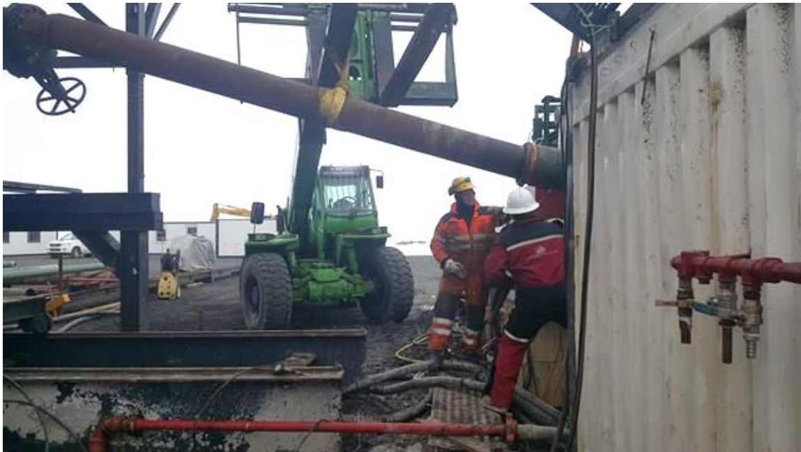
Figures 1-3. The drill crew working on connecting the flow-line.
