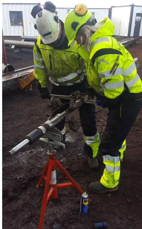
Figure 1. ÍSOR's logging engineers, Hörður and Valdís, preparing for CBL this morning.
