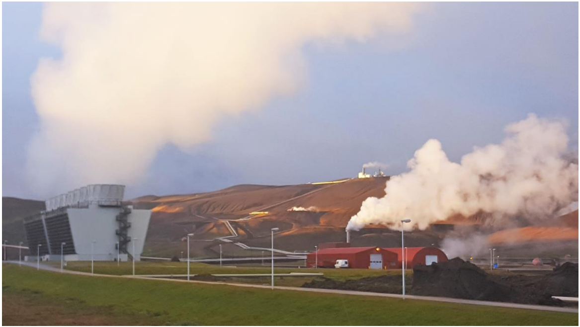
Figure 1. Picture showing the Krafla cooling towers in the foreground and the Sleipnir rig drilling well K-41 in the background.
