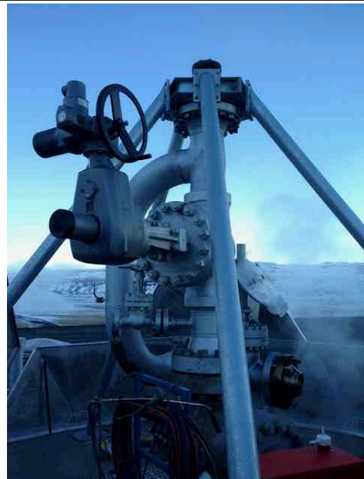
Photo 48: Wellhead valves
