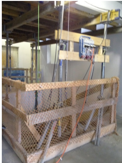
Photo 82: Temporary protection of stairwell
