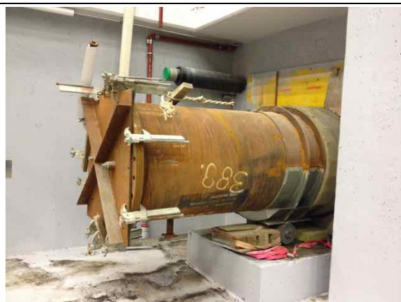
Photo 74: Steam supply pipe coming into powerhouse, with insulation
