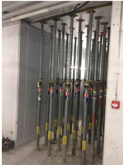
Photo 80: Supports in basement for heavy turbine transport above
