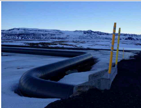
Photo 51: Steam supply line crossing road
