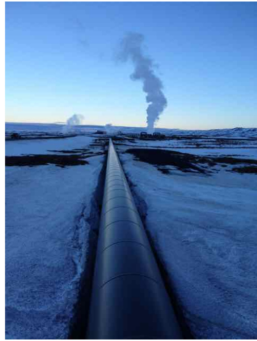
Photo 50: Steam supply line with powerhouse in background
