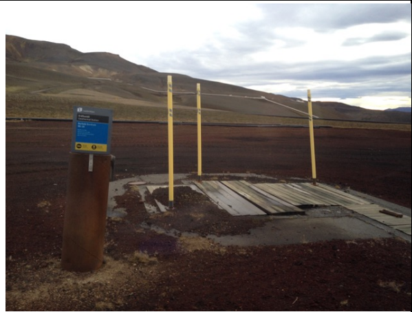
Photo 86: Closed wellhead from deep drilling project at Krafla
