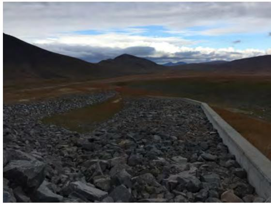
Photo 25: Concrete barrier between fuse plug and main part of Desjará dam
