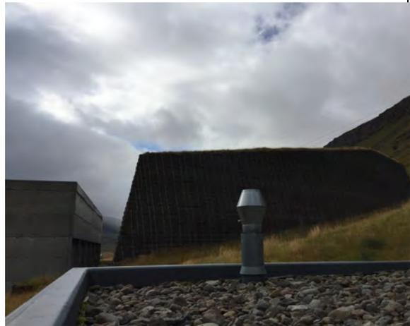
Photo 116: Switchgear house avalanche protection
