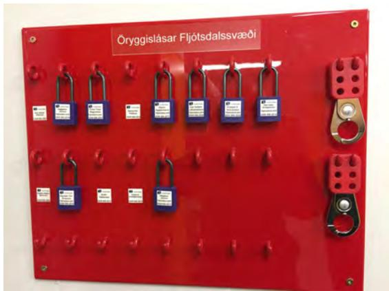
Photo 52: Individual safety locks for work on equipment in intake gate house
