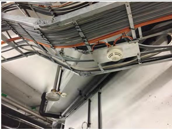
Photo 81: Fire detector and sprinkler on generator level
