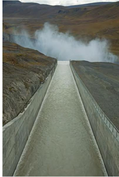
Photo 28: Kárahnjúkar spillway in operation
