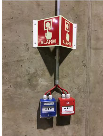
Photo 88: Flooding and fire alarms
