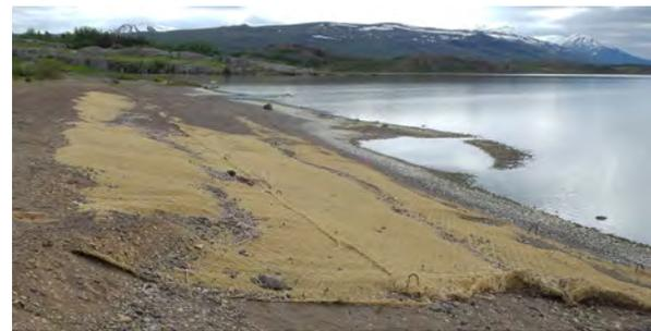
Photo 125: Bank-erosion protection on Lagarfljót lakeshore near Egilsstadir
