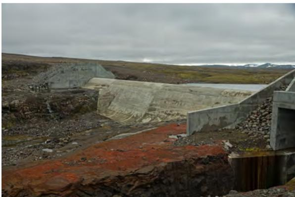
Photo 35: Grjótá overflow spillway
