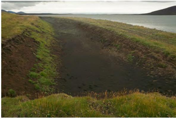
Photo 13: Sediment traps for wind-eroded material, eastern shore of Halslón
