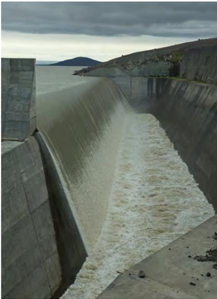
Photo 27: Kárahnjúkar dam ungated spillway
