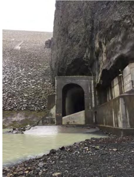
Photo 22: Bottom outlet lower end, Kárahnjúkar dam
