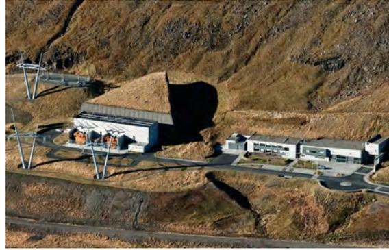
Photo 98: Aboveground buildings at Fljótsdalur power station (aerial photo: Landsvirkjun). From left to right: switchgear building, service building, workshop building, and access tunnel entrance
