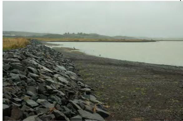
Photo 126: Bank-erosion protection on Lagarfljót lakeshore near Egilsstadir 2
