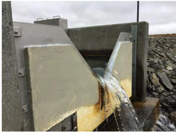
Photo 43: Kelduar dam seepage monitoring weir
