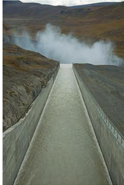
Photo 28: Kárahnjúkar spillway in operation
