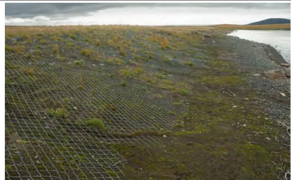
Photo 12: Bank-erosion protection on eastern shore of Háslón
