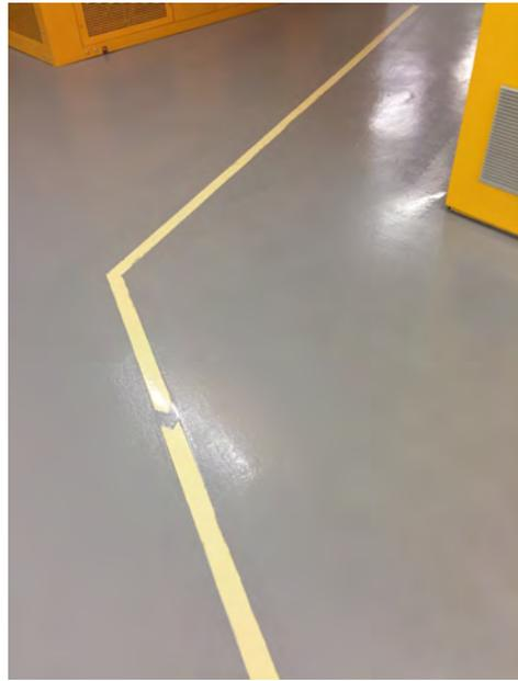
Photo 80: Reflective tape with escape route directions
