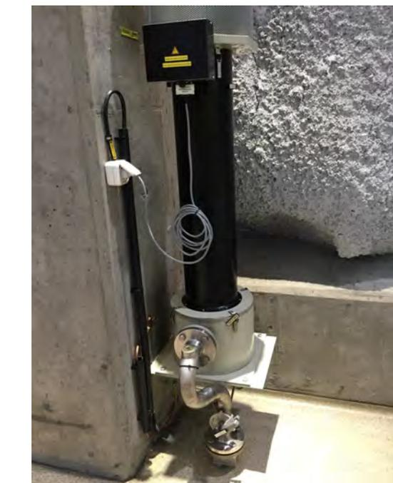
Photo 77: Air filters for oil mist in machine hall
