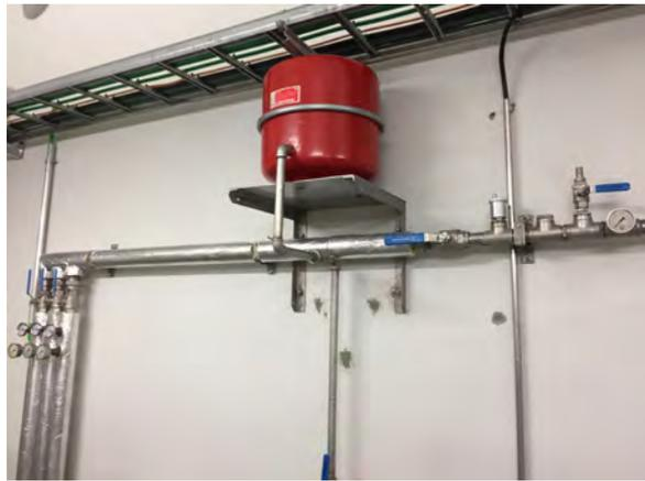
Photo 57: Heating system for Ufsarlón intake gate
