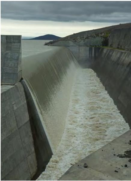
Photo 27: Kárahnjúkar dam ungated spillway
