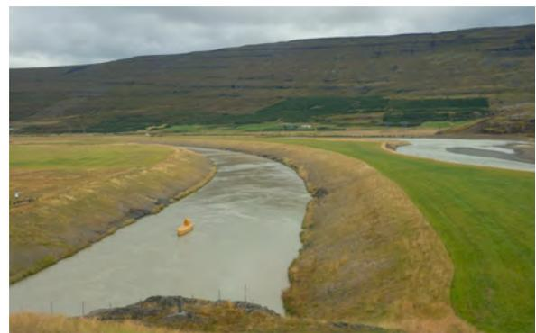
Photo 96: Fljótsdalur power station tailrace channel with art work
