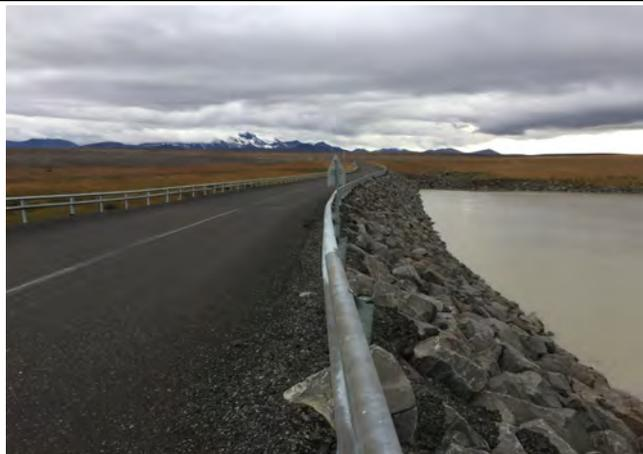
Photo 24: Fuse plug section of Desjará dam
