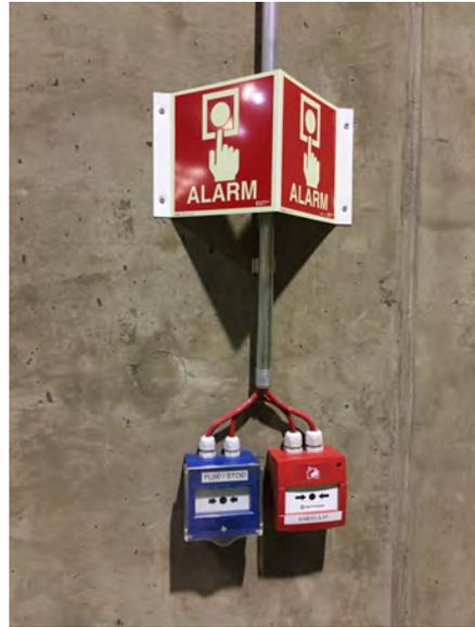
Photo 88: Flooding and fire alarms
