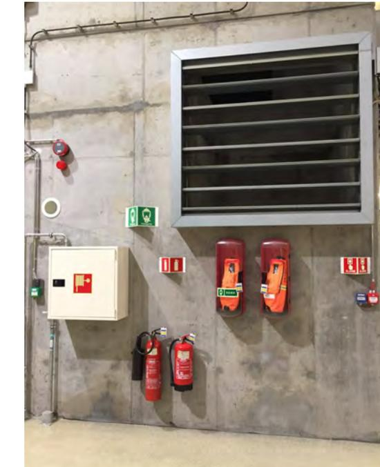
Photo 78: Ventilation, firefighting equipment, safety masks, alarms in machine hall
