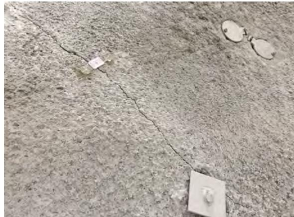
Photo 76: Rock bolts and instrumentation on machine hall wall
