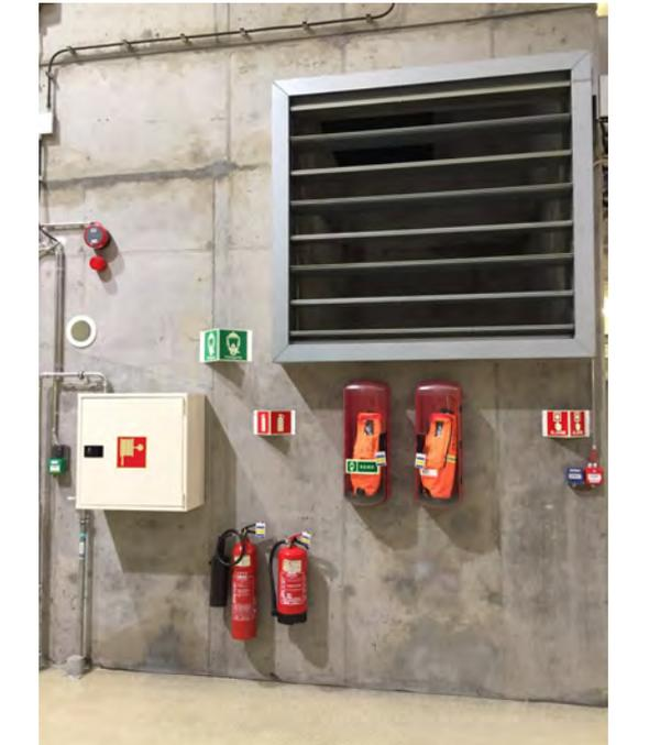
Photo 78: Ventilation, firefighting equipment, safety masks, alarms in machine hall
